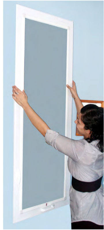
3. Push the screen completely into the frame
