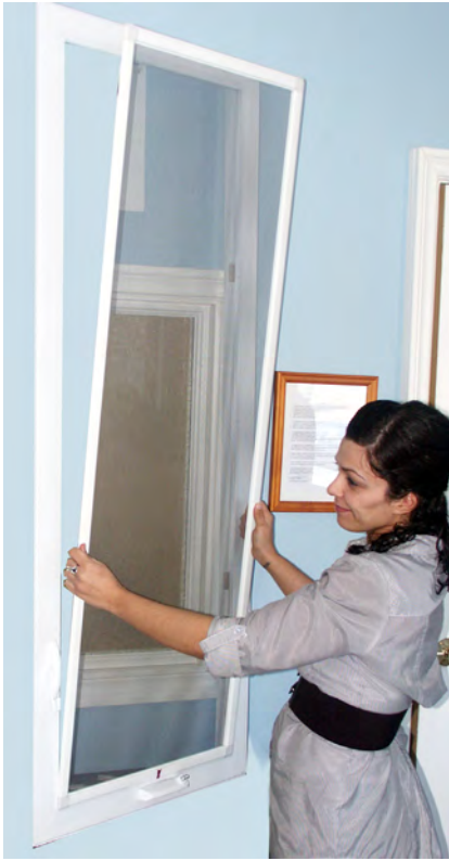
1. Lower the screen into the frame sill
